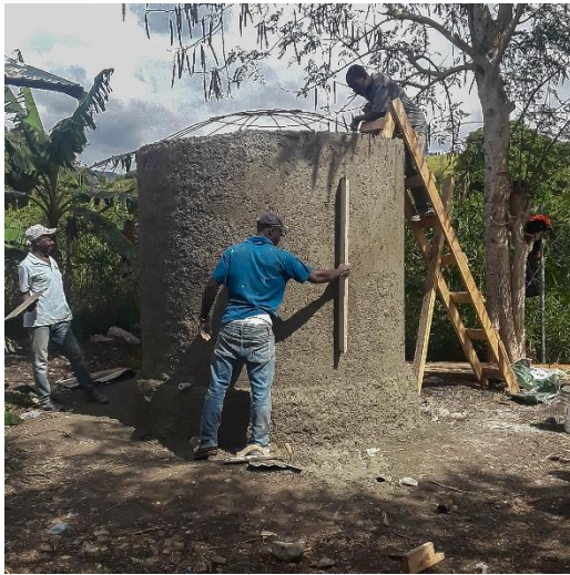
Masons constructing a 1,500-gallon cistern.
